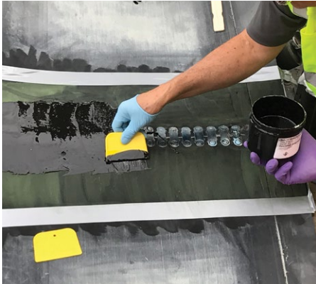
Before Metal Clips Splice Repair
