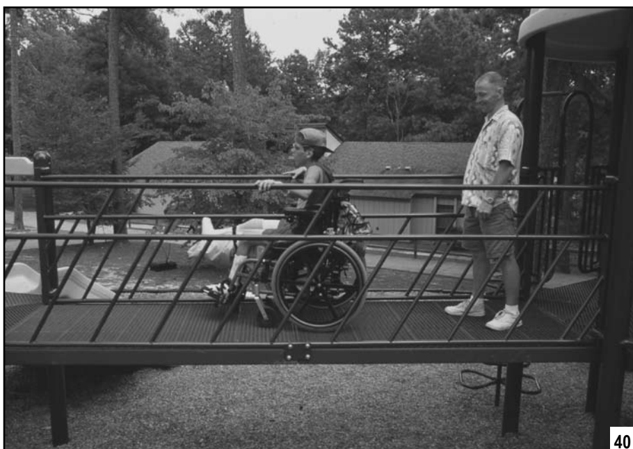
This photo illustrates an elevated accessible route:
